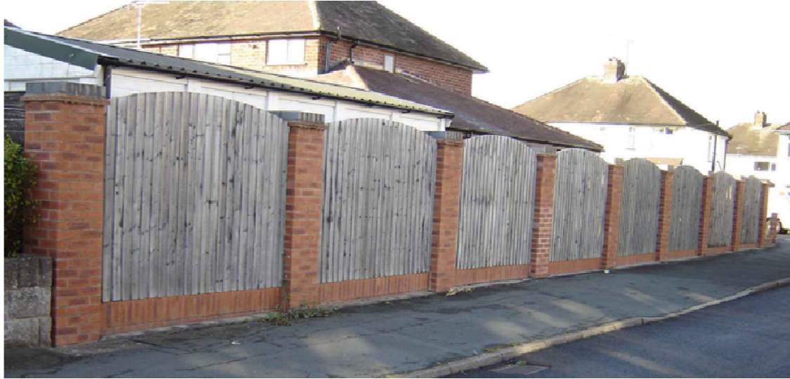
WALL WITH FENCE ABOVE
