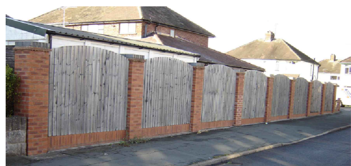
WALL WITH FENCE ABOVE
